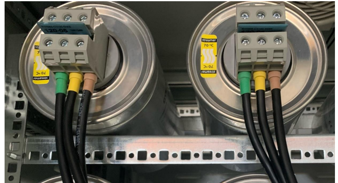
Installation of vFPTs on the capacitors
